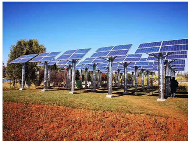
Solar Pumped Hydropower Station in Kunming Dagan Wetland Park
