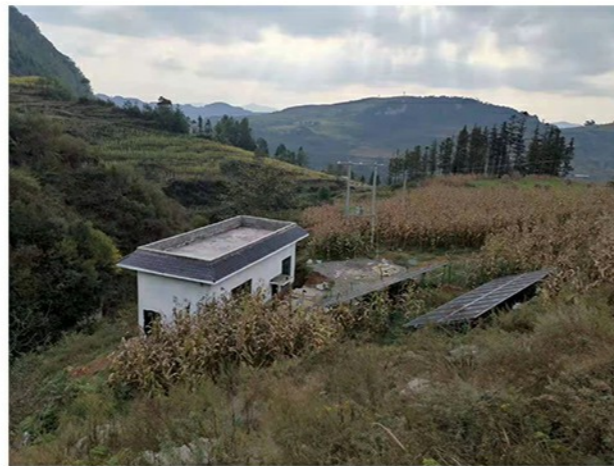
5.5KW PV+Grid Complementary System in Guizhou Province
